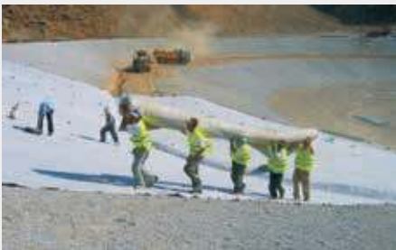
Landfill surface drainage/sealing
