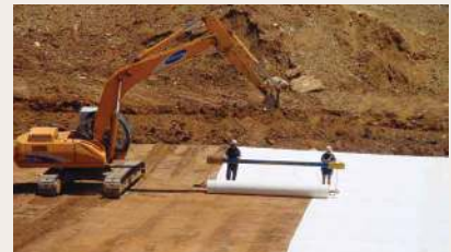
Laying Polyfelt® Enviromat GCL using crane.
