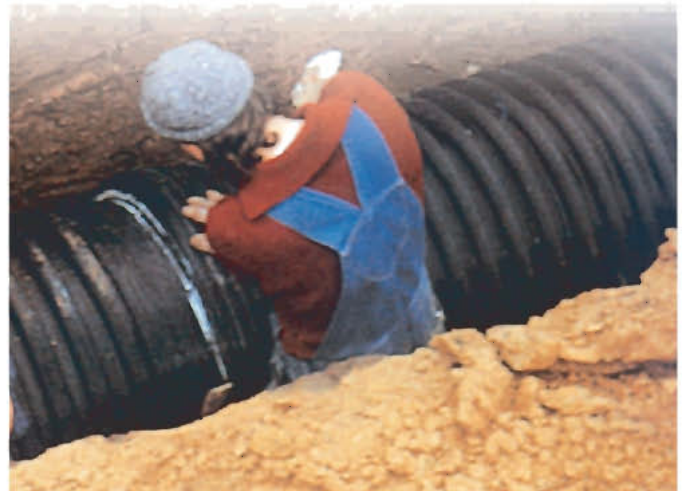
Socket-Gasket section of FKS pipes picture.
